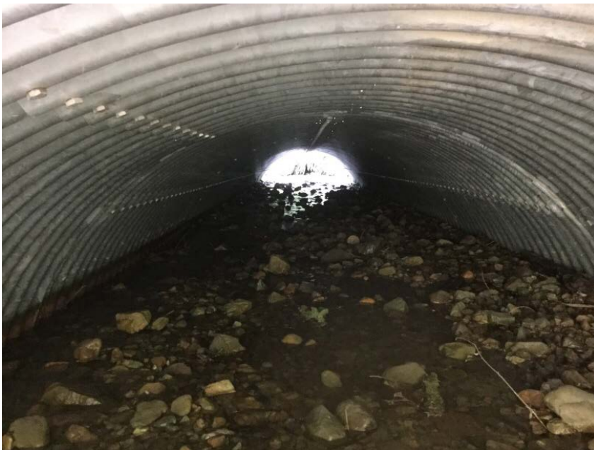
Looking through culvert
